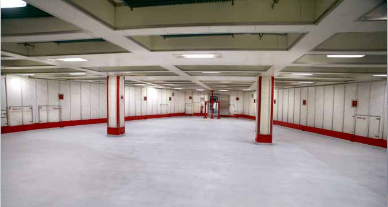
Completed cargo hold
